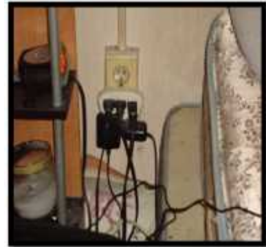
Unsafe Wiring
