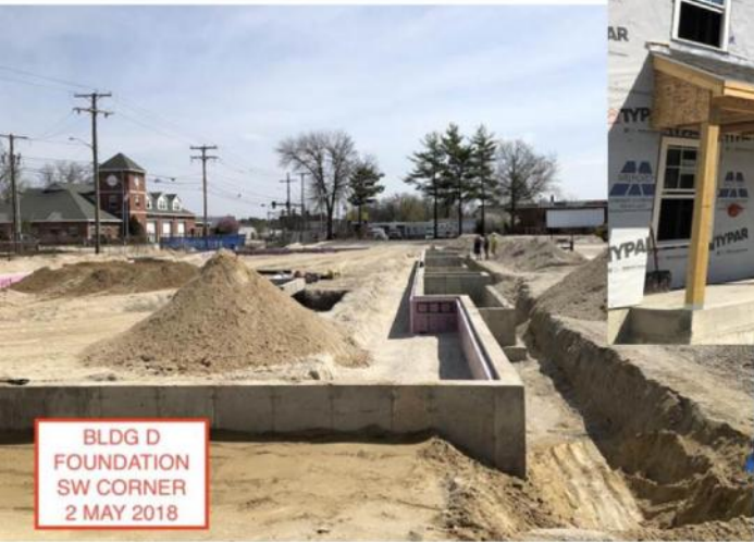
22 Marshall St in progress
