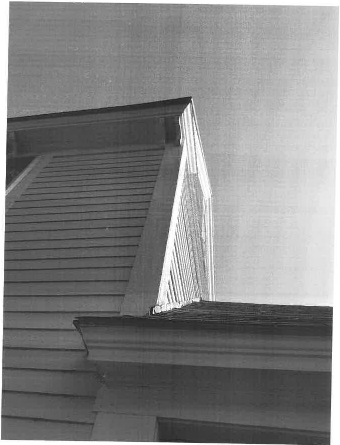
View of corner bracket ornamentation
