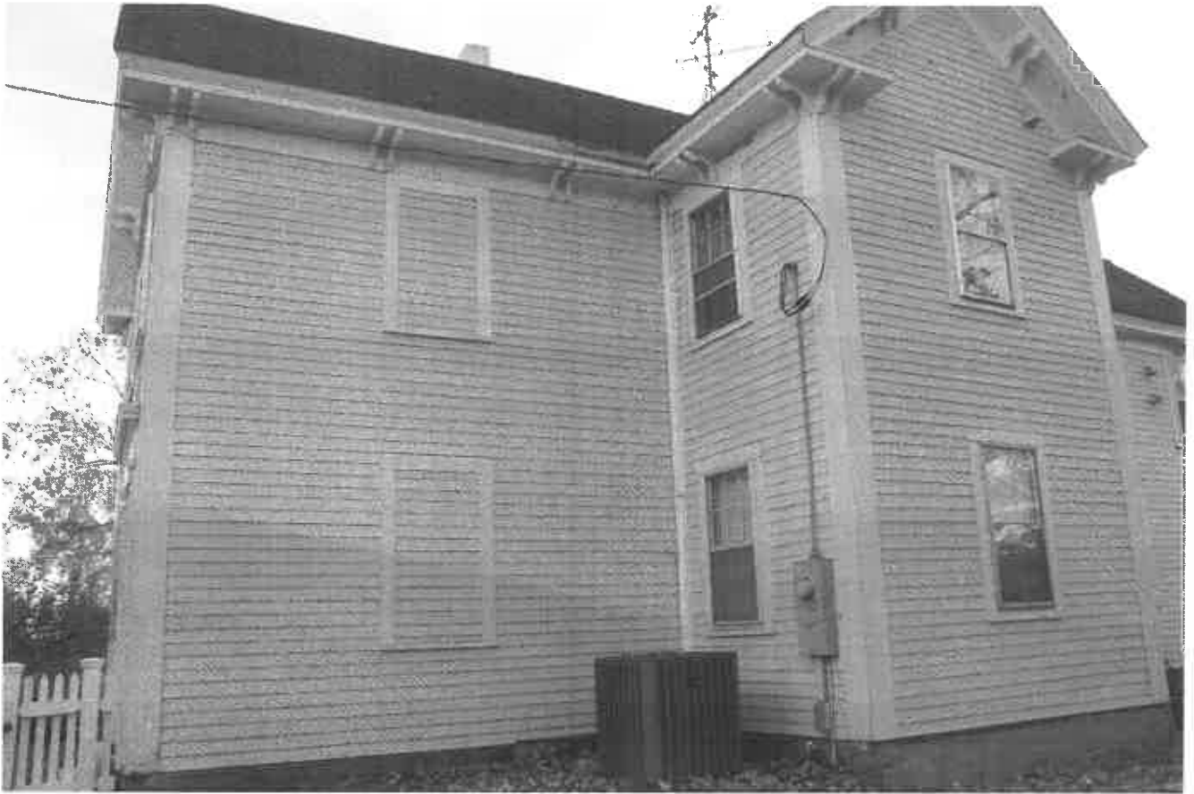
View of house from inside property near corner of the lot on Concord Street. Door would not be visible from here.
