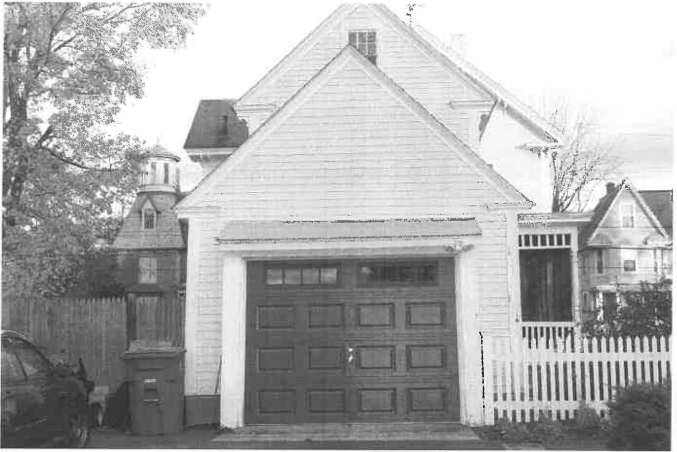
View of garage door - cannot see proposed door or landing from this view
