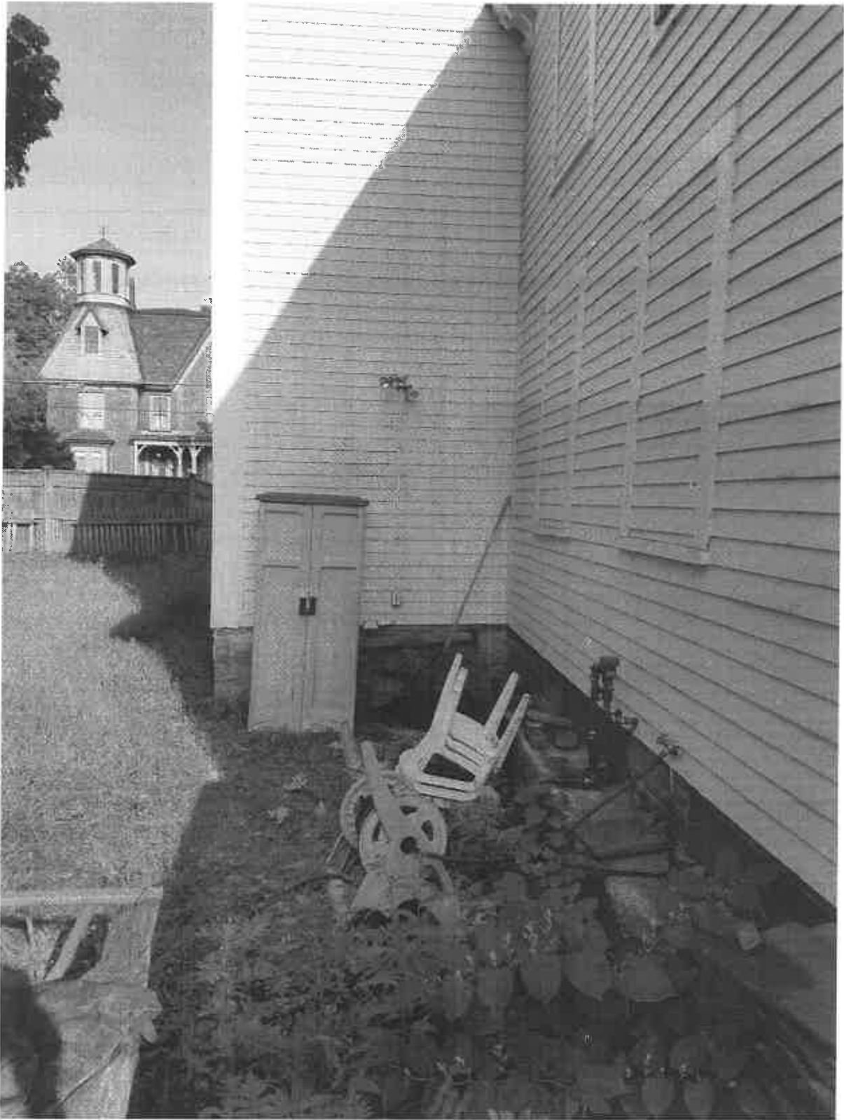
View of el and 6 foot tall fence along Concord Street
