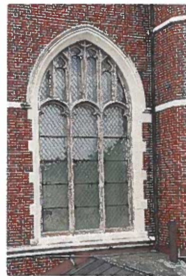
East Tower Window in 2023
